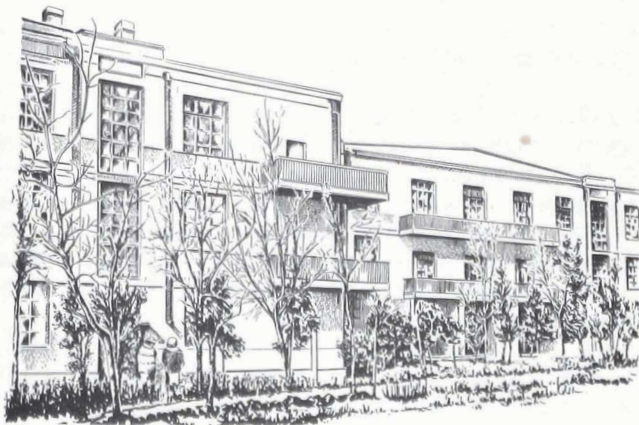
First three-storeyed blocks of flats in Stalinabad.
